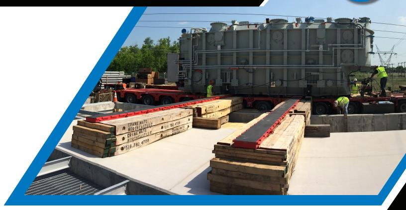
When space limitations and costs preclude the use of a crane, the Power Slide System delivers a simple, safe, and efficient way to move heavy and oversized loads of 50 to more than 2,000 tons! With rugged construction built to withstand daily use and extreme loads, the Power Slide is fabricated in-house to provide a quick turnaround of customized solutions. Features including integrated lifting, side shifting and leveling pads can be tailored to the application needs.
