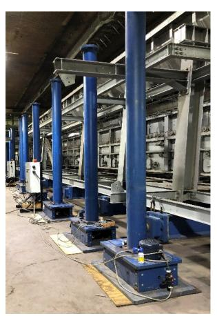
The modular lift system was rapidly assembled inside of the plant in just two days of double shifts. The system lifted the 138-ton conveyer into place and positioned it on grade with a total lift time of only 30 minutes. Tear-down was accomplished in a single day of double shifts.
