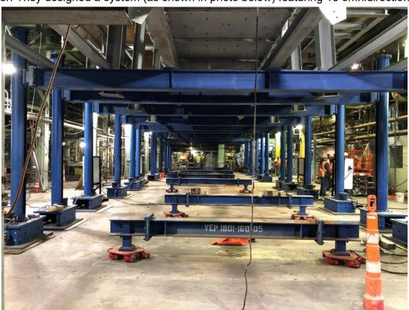
load skates each with a 10-ton capacity, and 12 custom-fabricated, 23-foot-long support beams, each with a 19-ton capacity. This solution enabled the company to translate the conveyer about 20 feet and position it on grade.
