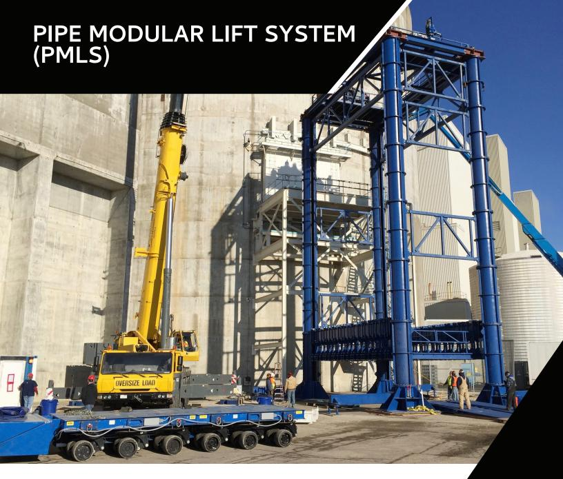
Engineered Rigging's patent-pending Pipe Modular Lift Systems (PMLS) eliminates the hazards of suspended loads. Different from all other heavy lifting systems, the PMLS employs a platform that mechanically raises and lowers heavy cargo via a system of vertical lift rods connected through gearboxes to electric motors. The heavy-walled steel lift secures both the cargo and platform, providing positive mechanical engagement 100% of the time.
