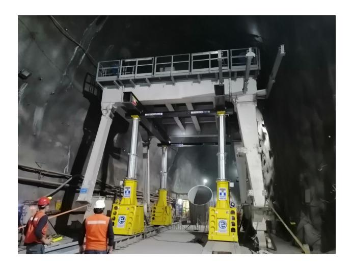
With a capacity of 337 tons at its maximum height, the SBL500 safely supported the 80-ton crane while the crane's legs were removed. The crane was then lowered and trolleyed out of the tunnel on the gantry. The gantry's trolley capabilities allowed us to move the crane 23 meters through the tunnel to the exit. Once outside of the tunnel, the crane was safely dismantled at ground height.
