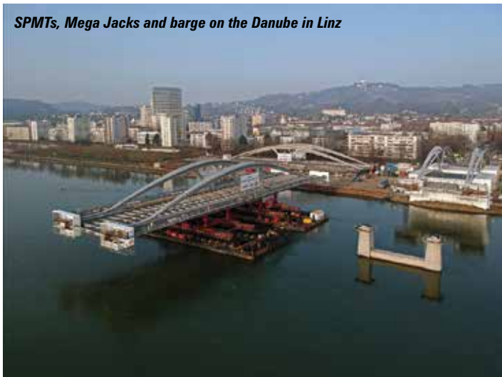
The 50 metre bridge section for the new Seibert Bridge is loaded onto the barge
