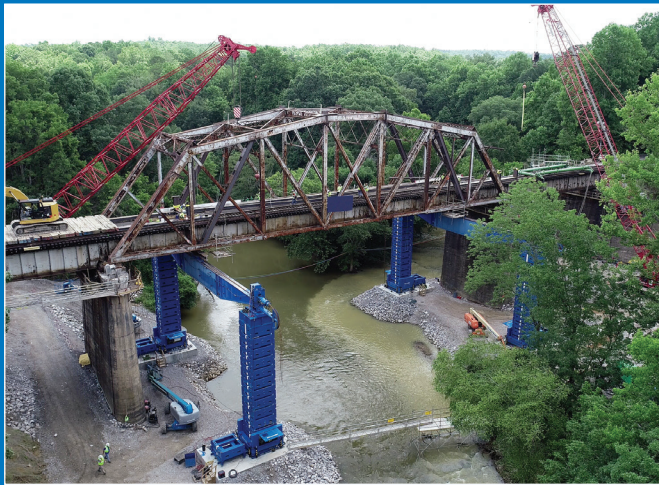
Accelerated Bridge Construction & Demolition
